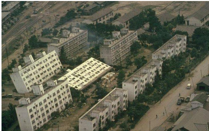
Figure 2.9 - Loss of Bearing Capacity due to Soil Liquefaction from Niigata, Japan 1964 Earthquake (Niigata Earthquake, 1964).
