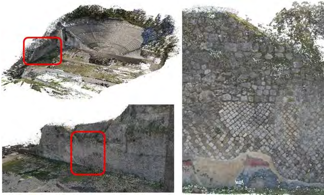
Figure 6: Detail of the point cloud of the theater wall.
