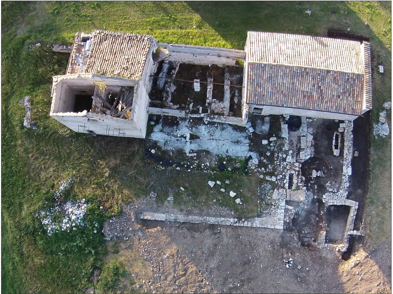
Fig. 5. Piana San Marco, aerial view of the excavation.
