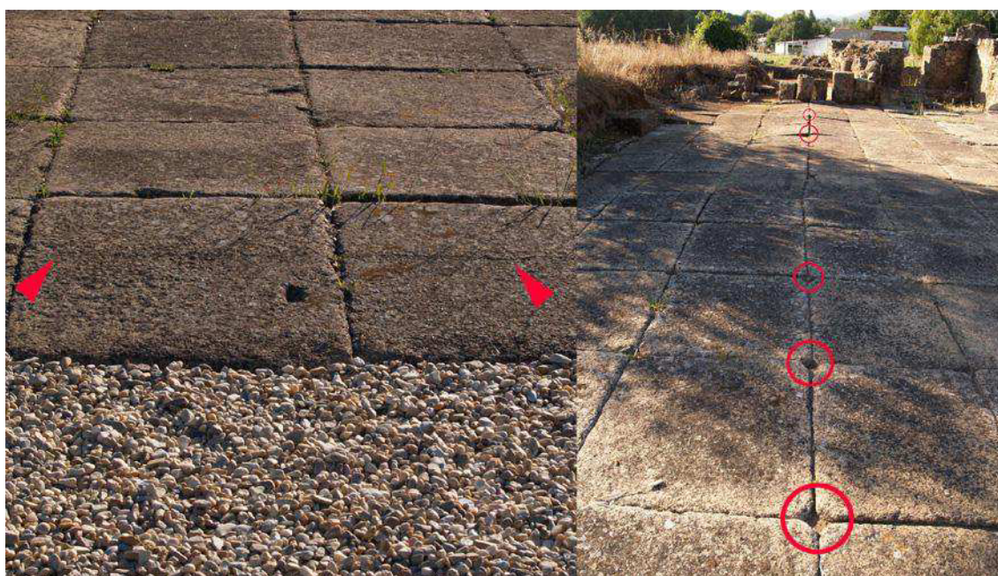
Fig. 9 – Left: Marks of heavy structures. Right: Holes in regular distance (© 7reasons).
