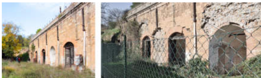
Fig. 6 - Fort Monte Antenne. The troop quarters front in two comparative photographs (2021–2024). Source: created by the authors.
