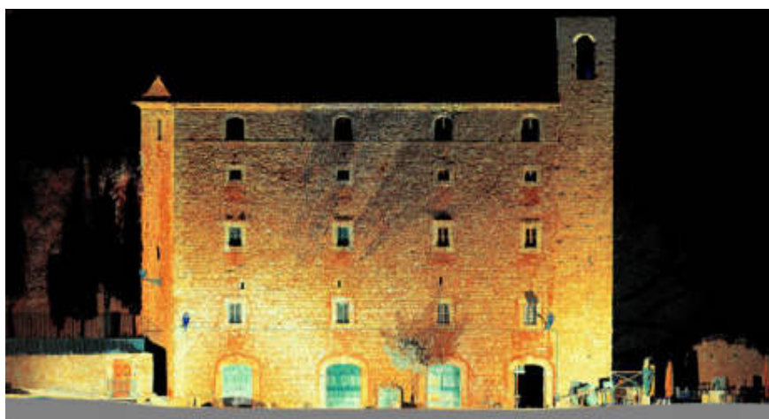
Fig. 1 – An image of the point cloud restitution of the Girifalco Fortress in Cortona. The reflectance highlights the heterogeneity of the masonry structures, highlighting the perceptive behavior and the characteristics of the surface alterations. Source: created by the authors.
