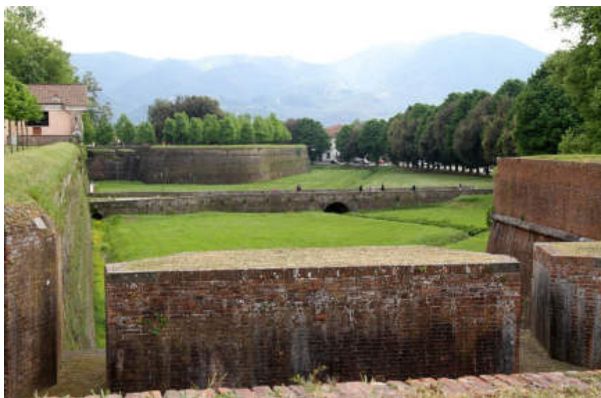
Fig. 6 – City walls of Lucca (LU). You can notice the architectural-constructive features that constitute the walls and their state of conservation (Source: www.comune.lucca.it/vivere-il-comune/luoghi/le-mura-di-lucca-un-parco-urbano/ ).
