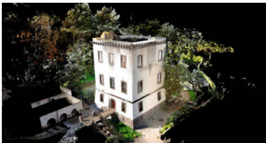
Fig. 2 – Ischia, Torre Guevara, restitution of the laser scanner survey of the exterior and contextual data. Source: created by the authors.
