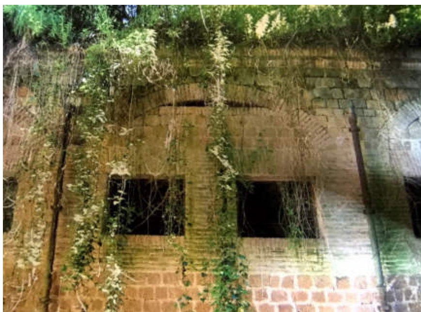
Fig. 3 - Roma, Forte Antenne, Paramento murario in tufo e mattone. (Source: created by the authors)
