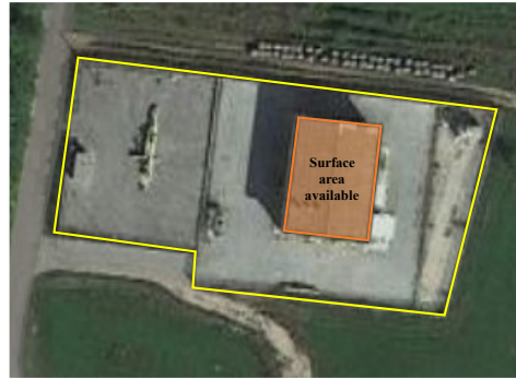
Figure 8.6. Layout of the RMS, with the surface area available for PV panels installation highlighted in orange colour.
