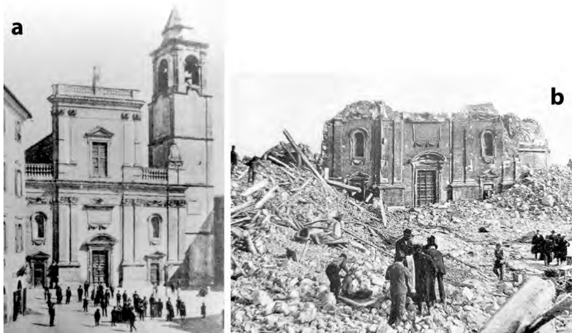
Fig. 11 Avezzano, church of San Bartolomeo (16th–17th century) before (a) and after (b) the 1915 earthquake (historical photos from personal archive of F. Galadini)
