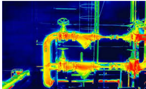
Figure 2.1: General representation of the results obtain trough the thermographic instrumentation.
