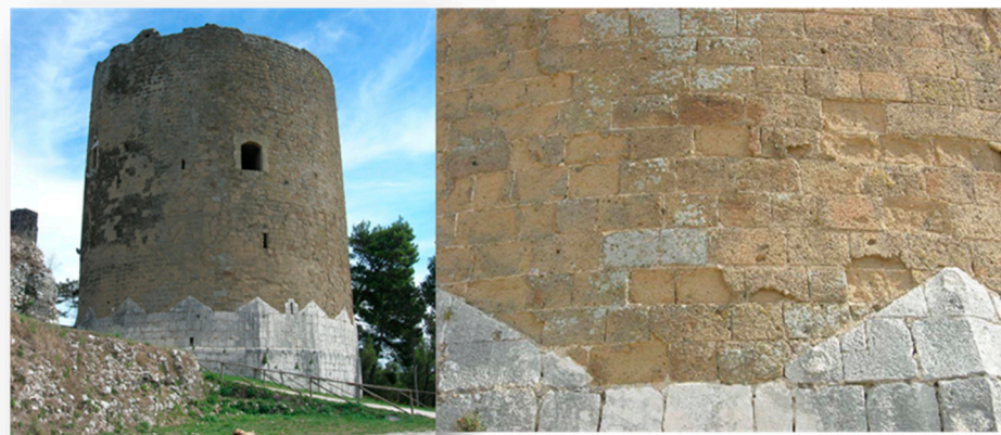
Figure 12. Example of the moderate physical weathering of facia vista Campanian Ignimbrite dimension stones (Mastio of the Caserta Vecchia Castle, Caserta Vecchia, left: whole building, right: physical weathering; picture by A. Langella).
