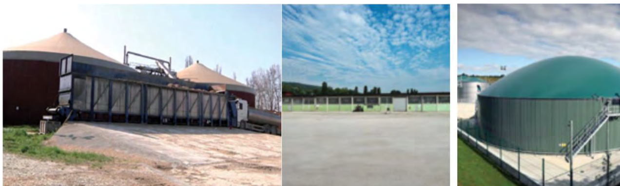
Figure 5. Iraci Borgia biogas plant.
