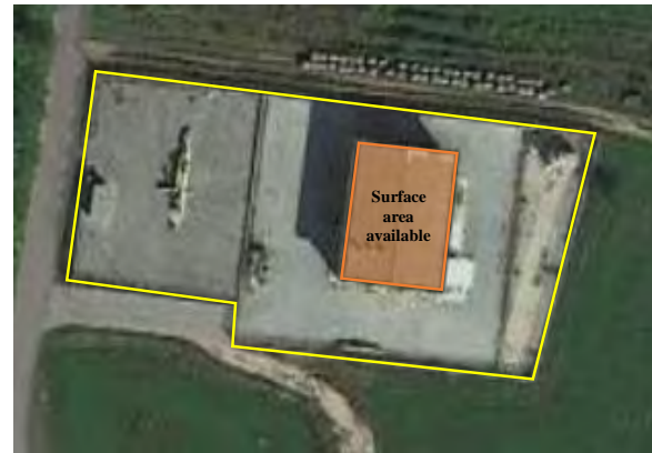
Figure 4. Layout of the RMS, with the surface area available for PV panels installation highlighted in orange colour.
