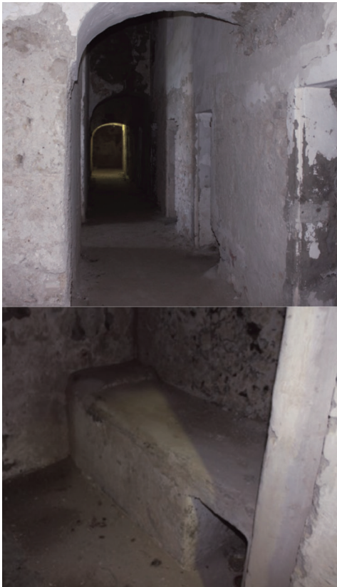
Fig. 7- Bourbon cells. Pictures of the narrow hallway and the stone beds and pillows (photos by the authors)
