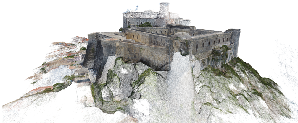
Fig. 5- Photogrammetric survey from a drone of the Angevin castle that highlights its mammoth architectural structure (graphic elaboration by the authors)
