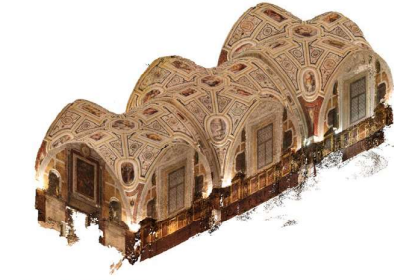
Fig. 2. Digital photogrammetric model of the sacristy and description of the iconographic apparatus of the central vault. Graphic elaboration by the authors.
