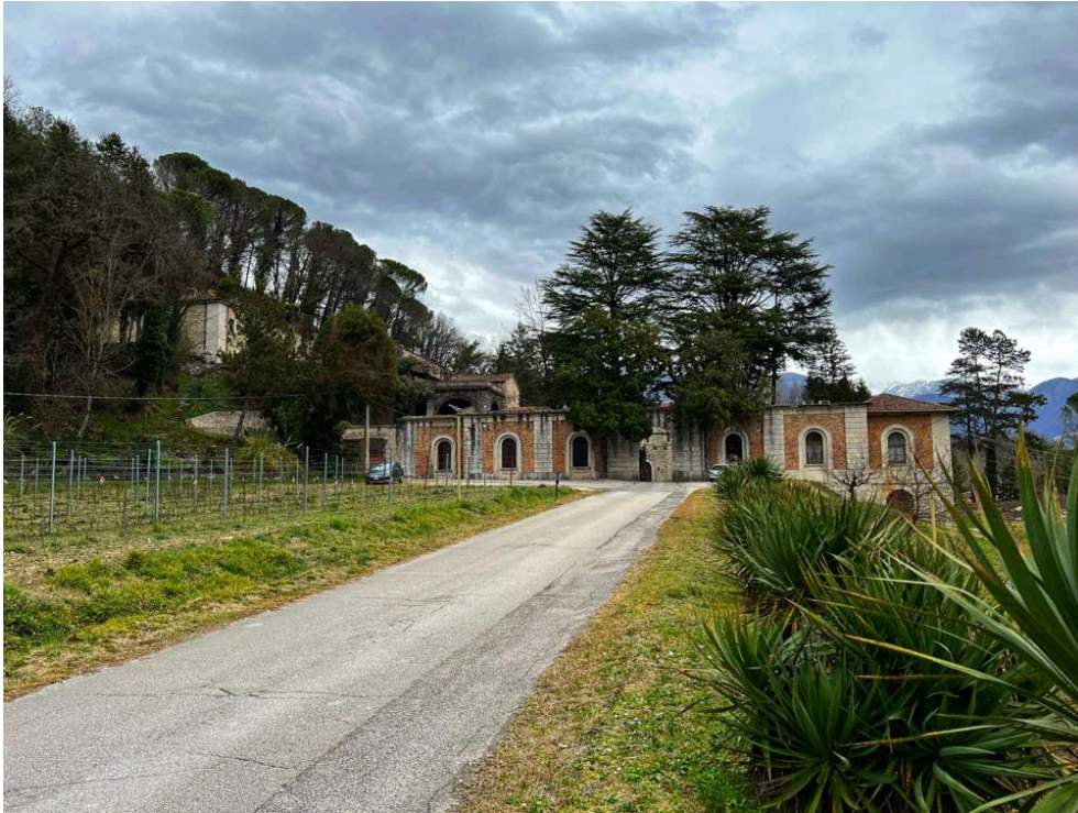
Figure 6. Atina: old steel mill re-functionalized as a winery.
