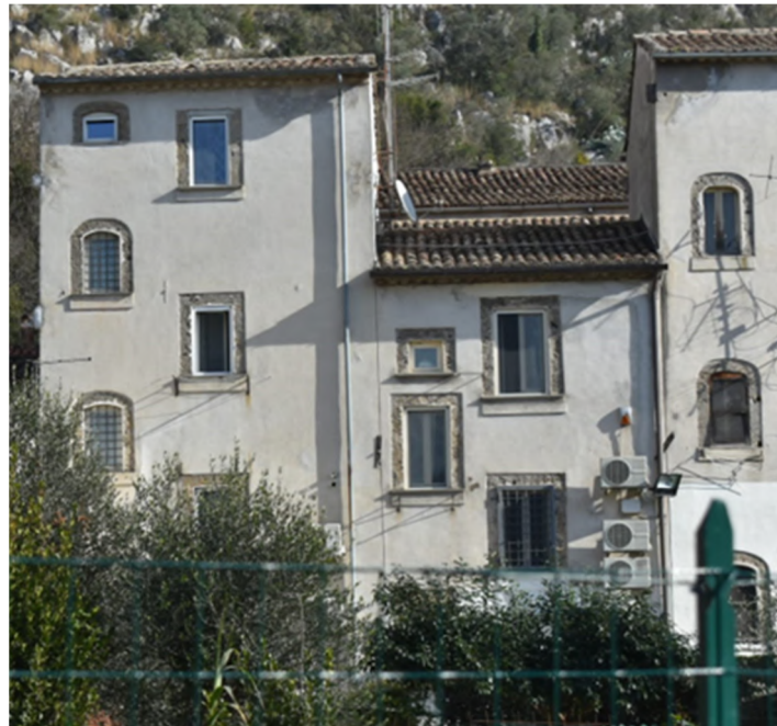
Figure 5. Example of building aggregate with S.U.s having different numbers of stories and staggered slabs.
