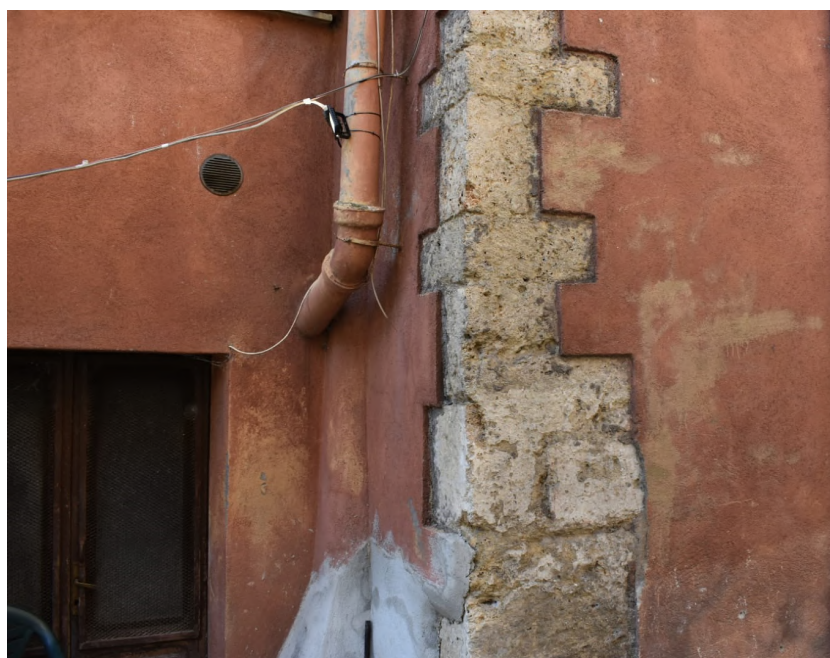
Figure 13. Square blocks at the corner of the ground story.
