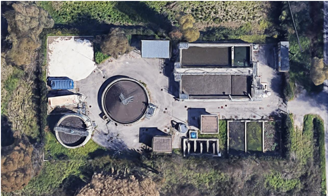
Figure 52 Wastewater treatment plant, BorgoPiave Latina.
