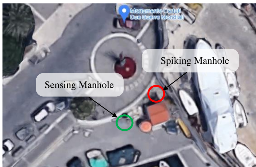
Figure 68 Anzio Monumento Caduti Due Guerre Mondiali real test location. The red circle indicates the spiking manhole, while the green is the sensing one. The manholes were located 10 meters apart.
